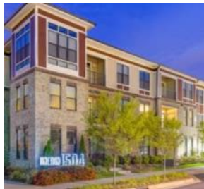
Junction 1504 Apartments Residential Charlotte, NC
