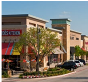
Alliance Towne Center Retail Fort Worth, TX
